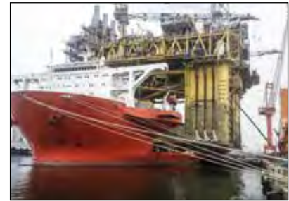
Synchronous superlift and launch
