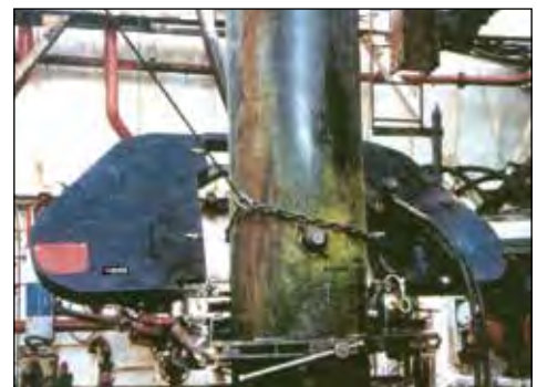
▼ Decommissioning job with band saw.
