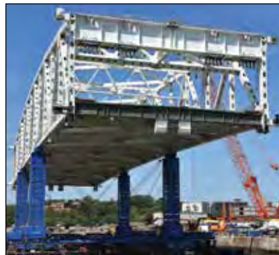
▼ Enerpac Jack-Up System hoists 1500-ton span on Fore River Bridge.
