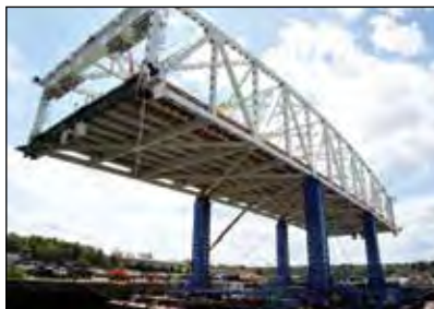
Incremental bridge lifting
