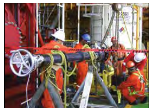
▼ CHT2000 hot tapping offshore application.
