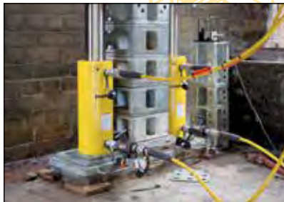
Bridge lifting and launching
