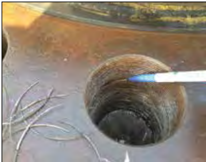
▲ A typical thread before refurbishment
