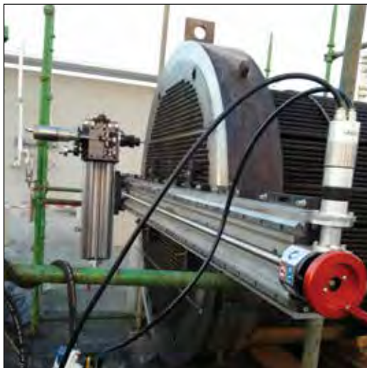
▼ MRY Milling machine on a heat exchanger.
